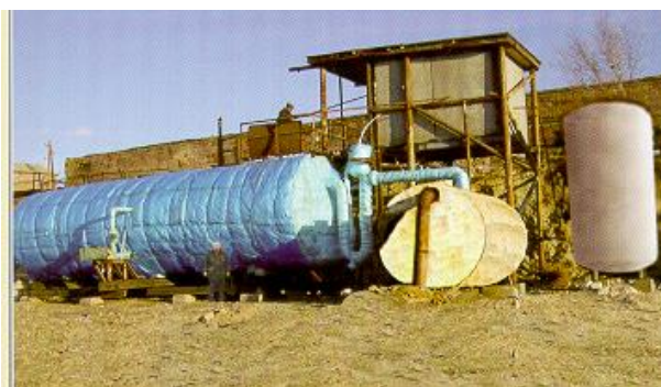
Figure 14. Biogas plant in Bartsrashen, Armenia (bioreactor 52m 2 )
